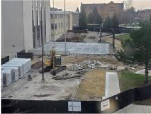
South Entrance Excavation
