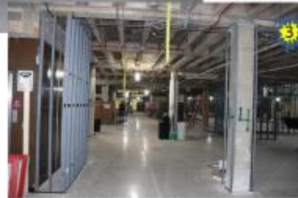
East-West corridor view
