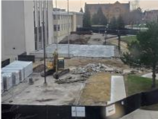
South Entrance Excavation
