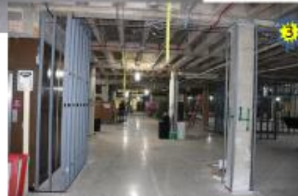
East-West corridor view
